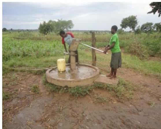
**Figure 1: A poorly maintained shallow well with a cracked apron**
